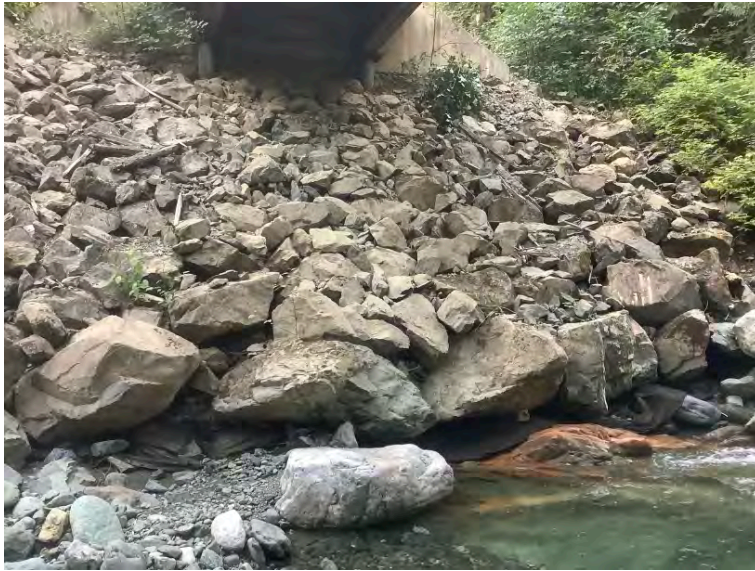
Right Bank Abutment when facing downstream
