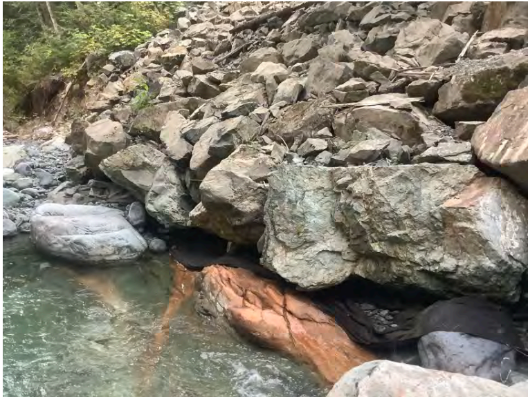
Right Bank Abutment when facing downstream
