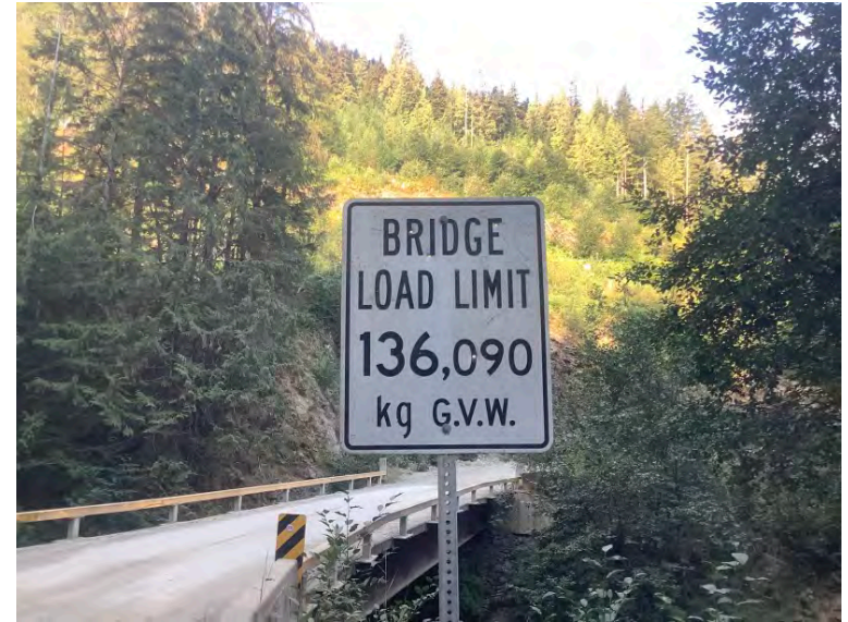
Load Rating Sign
