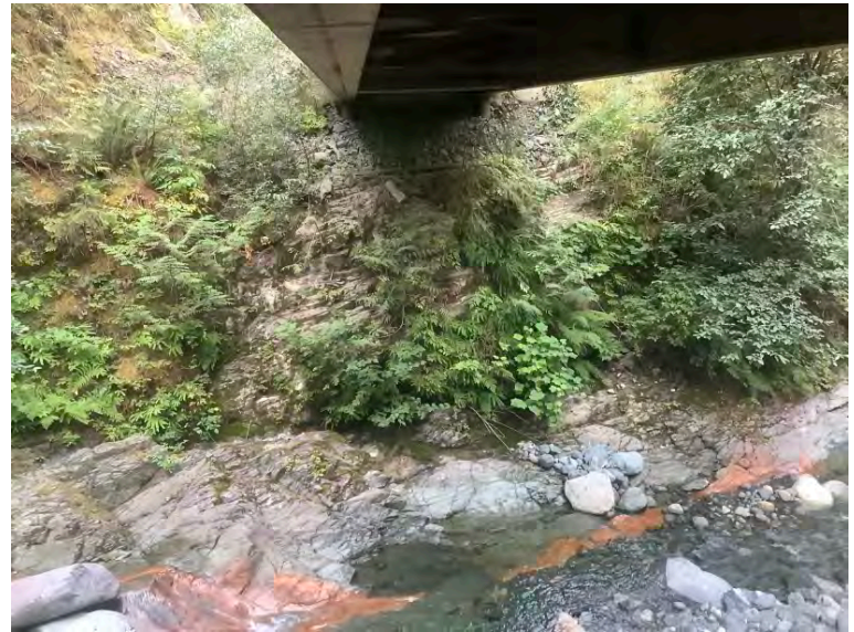
Left Bank Abutment when facing downstream
